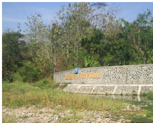
Figure 15 . DAM Check Building
