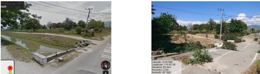
Figure 2. Gumbasa canal at the crest of Petobo slide footprint, before (left) and after (right) the 2018 earthquake (Kusumawardani et al., 2021).
