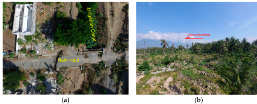
Figure 9. Photos showing GS and LS morphological features observed at Petobo sliding area: (a) ground slide (GS), (b) liquefaction spread (LS).
