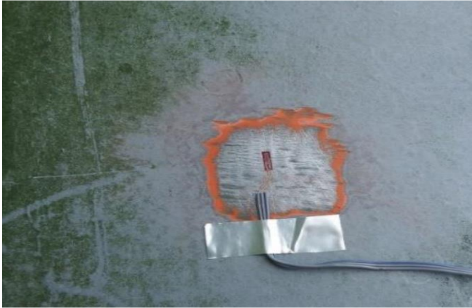
Figure 6. Placement of conventional strain gage on the flange of diagonal frame.
