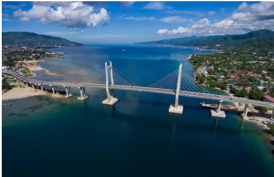
Figure 1. “Merah Putih Ambon” cable-stayed bridge.
