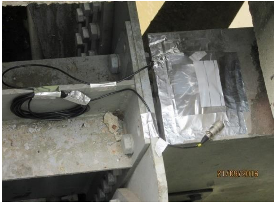
Figure 8. Placement of accelerometer on the cross beam of the monitored bridge.
