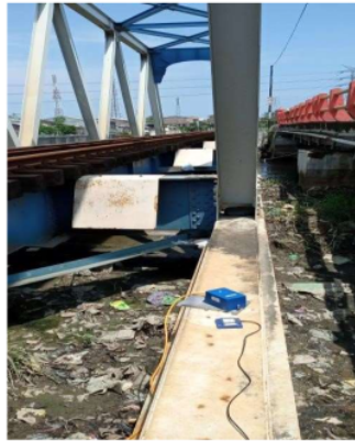
FIGURE 2 Sensor accelerometer placed at the bridge's structure with X facing the east.
