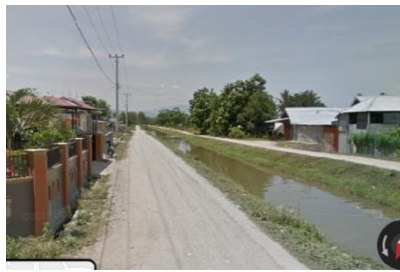
Photo 1. Before EQ (looking S)
