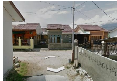
Photo 10. Before EQ (looking SW)
