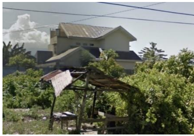
Photo 9. Before EQ (looking SE)
