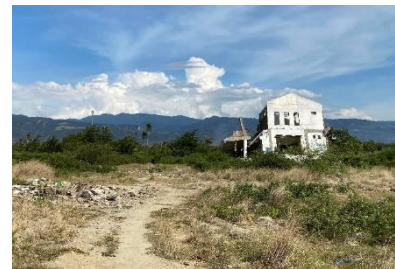
Photo 7'. After EQ (looking E)
