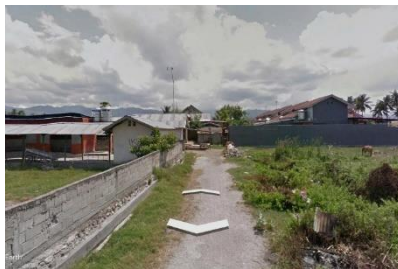
Photo 11. Before EQ (looking E)
