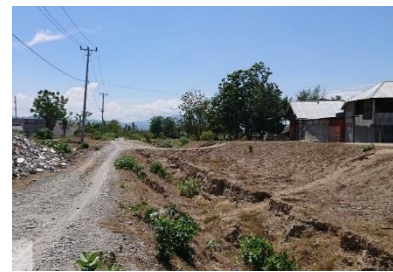
Photo 1'. After EQ (looking S)
