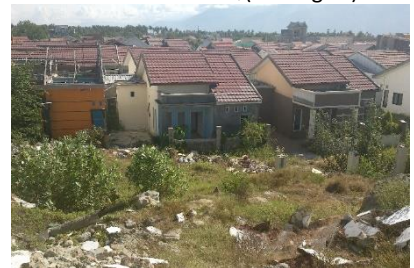
Photo 10'. After EQ (looking SW)
