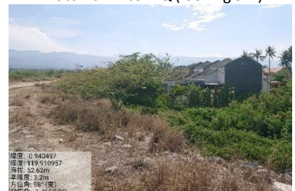
Photo 11'. After EQ (looking E)
