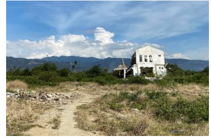
Photo 7'. After EQ (looking E)
