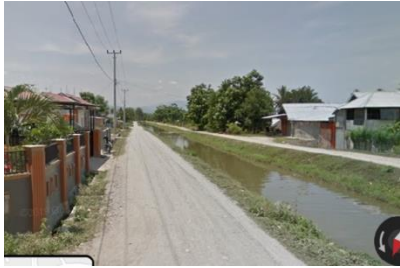
Photo 1. Before EQ (looking S)
