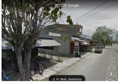
Photo 8. Before EQ (looking W)
