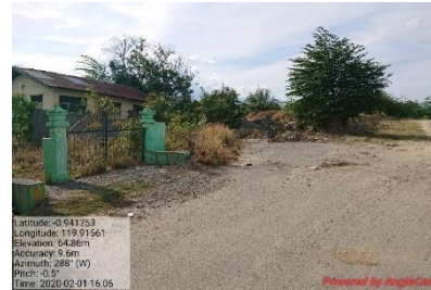
Photo 12'. After EQ (looking NW)
