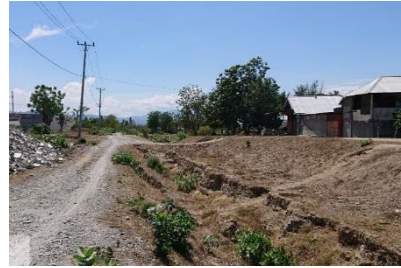
Photo 1'. After EQ (looking S)
