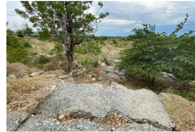
Photo 4'. After EQ (looking SW)
