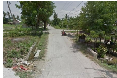
Photo 4. Before EQ (looking SW)
