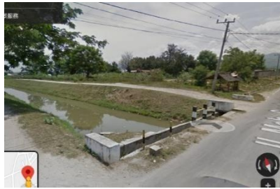
Photo 2. Before EQ (looking NE)
