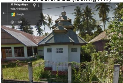
Photo 6. Before EQ (looking E)
