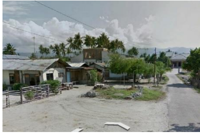
Photo 7. Before EQ (looking E)
