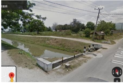
Photo 2. Before EQ (looking NE)
