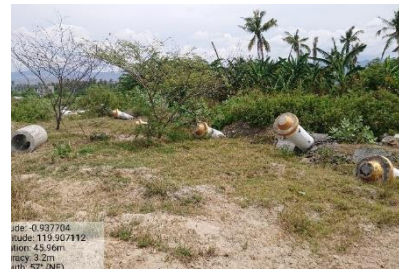
Photo 5'. After EQ (looking W)
