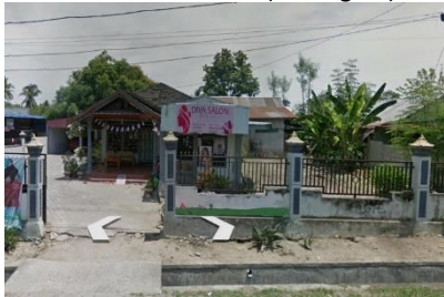
Photo 3. Before EQ (looking N)
