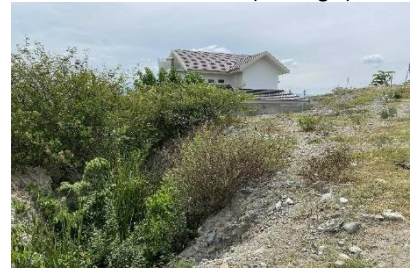
Photo 9'. After EQ (looking SE)
