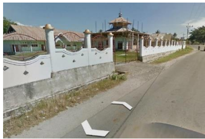
Photo 5. Before EQ (looking NW)
