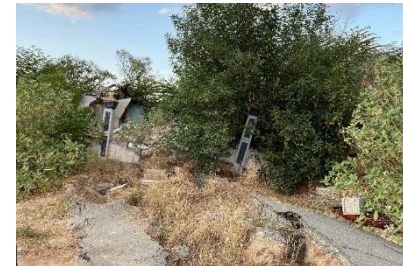
Photo 3'. After EQ (looking N)
