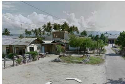
Photo 7. Before EQ (looking E)
