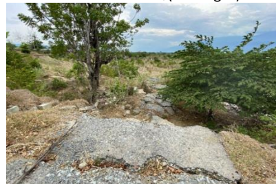
Photo 4'. After EQ (looking SW)
