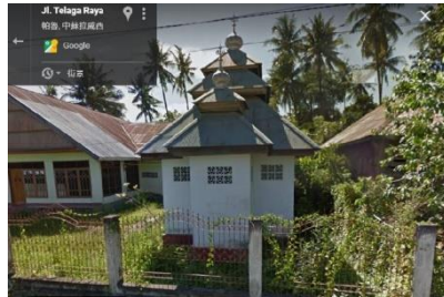
Photo 6. Before EQ (looking E)
