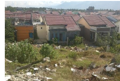
Photo 10'. After EQ (looking SW)
