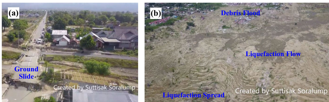
Fig. 18 Morphological features observed from the snapshots of drone videos by Soralump (2018). a Photo of the ground slide feature along Moh. Soeharto road to the east boundary of Petobo slide (facing east). b Photo of the features of liquefaction spread, liquefaction flow and debris flood on the south-eastern portion of Petobo slide (facing west)
