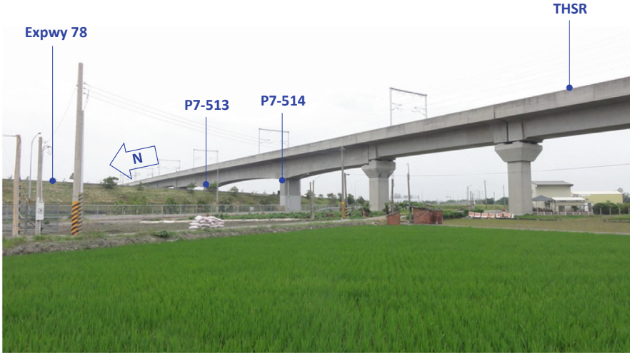
Fig. 4. Intersection of THSR and Expwy 78 Embankment (viewing NE).
