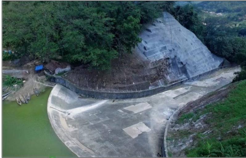
Figure 1. Construction of the spillway and chute spillway of the Cacaban Dam
