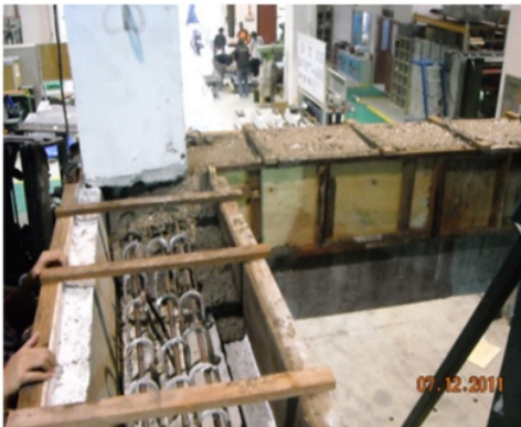
(a) construction of in-plane and out-of-plane beam and top column
