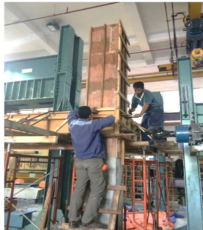
(b) construction of corner beam-column joint
