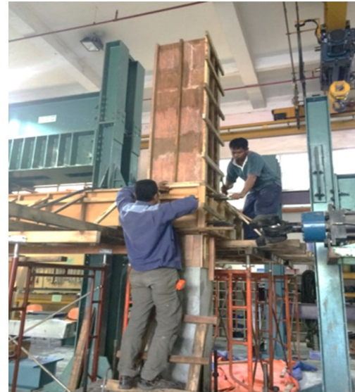
(b) construction of corner beam-column joint
