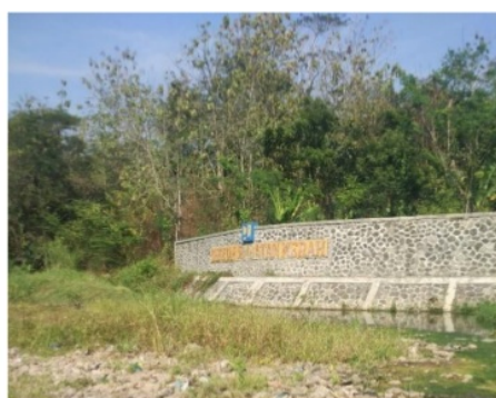
Figure 15 . DAM Check Building
