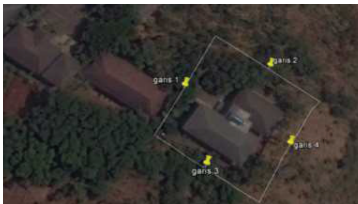
FIGURE 2. The location of landslide study on Universitas Negeri Semarang area
