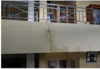
FIGURE 1. Some failure of beam and wall in Domestic Welfare Science Home Economics Department, Universitas Negeri Semarang
