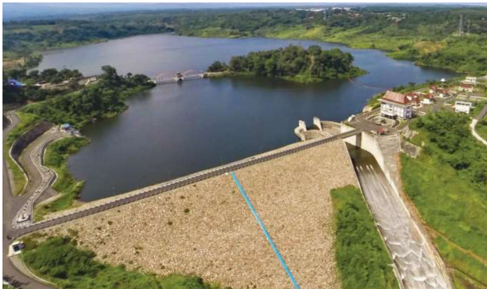
FIGURE 1. Reservoir and spillway at the Jatibarang Dam in Semarang
