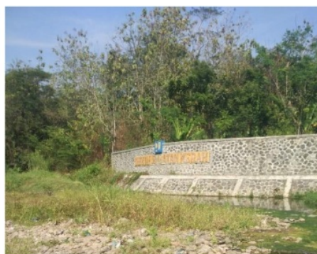
Figure 15 . DAM Check Building
