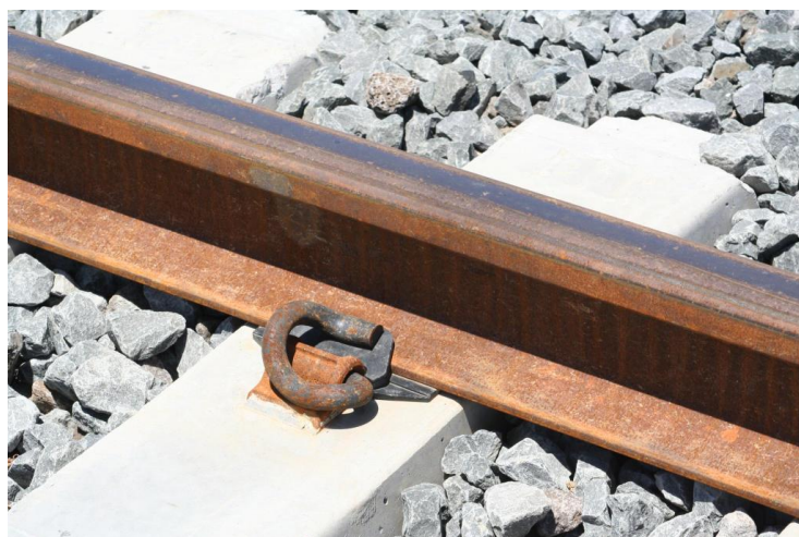
Gambar 2.9 Penambat tipe E-clips
