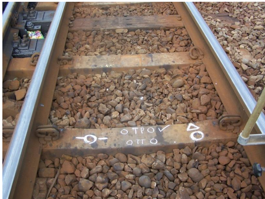
Gambar 2.11 Penambat tipe DE-clips
