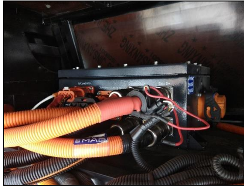
Gambar 2.6 High Voltage Control Box
