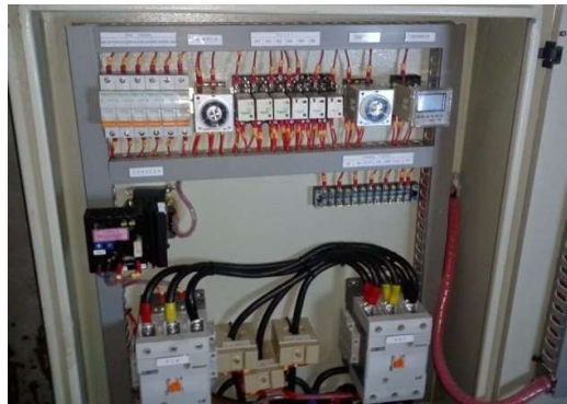
Gambar 4.31 Generator Set (Auto Switch System) Sumber: sariling
