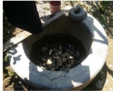
Figure 5. one of the well that could not be able to use anymore because of seawater contamination.
