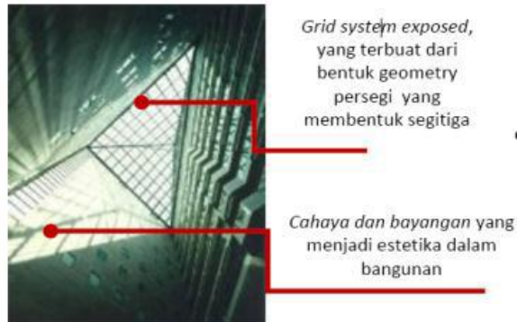
Gambar 2.51 Guggenheim Pavilion, The Mount Sinai Medical Center Expansion & Modernization (1992) Sumber : www.pcfandp.com
