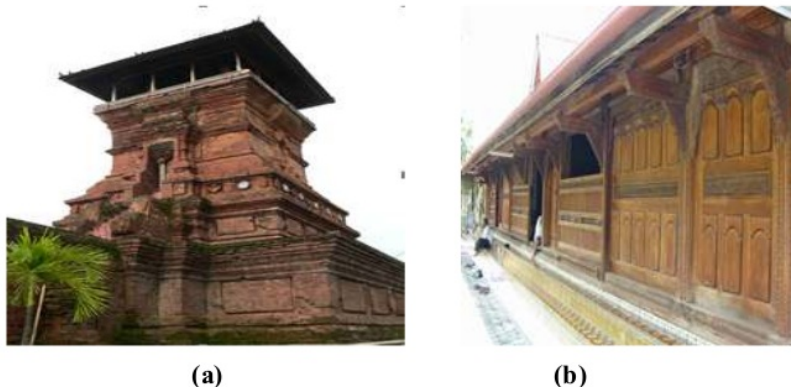
Figure 2. Traditional buildings in Kudus which are full of ethnomathematics; (a) the Mosque of Menara Kudus, (b) the traditional house.
