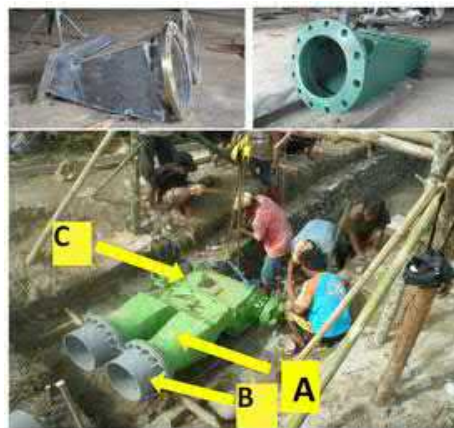
Gambar 2.13 Inlet Adapter
