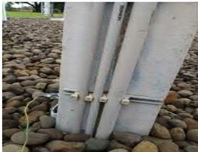
Gambar 3.8 Grounding Leakage Current Monitor Sumber : (Nur Amelia, 2017)
