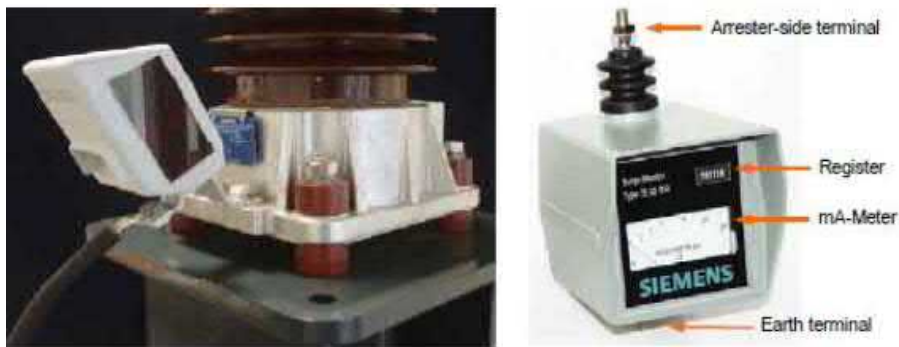
Gambar 3.1 Peralatan monitoring dan insulatorudukan Lightning Arrester Sumber : (Rizaldy, 2017)
