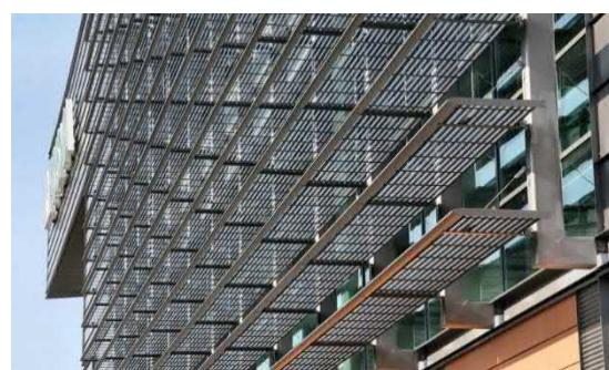
Gambar. 5.7. Sun shading
