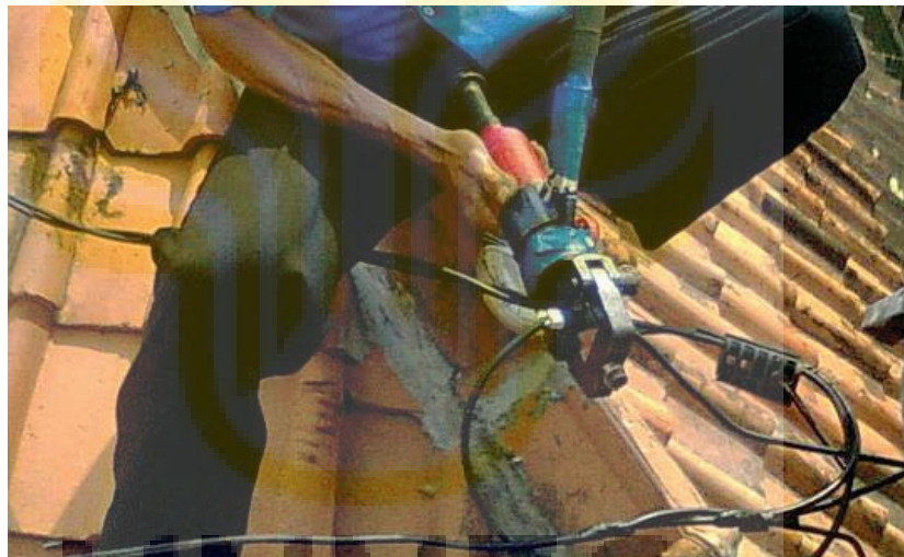
Gambar 2.13 Pemasangan Compression Connector
