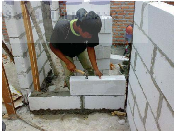
Gambar 5.4 Dinding Bata Hebel Sumber : https://sites.google.com
