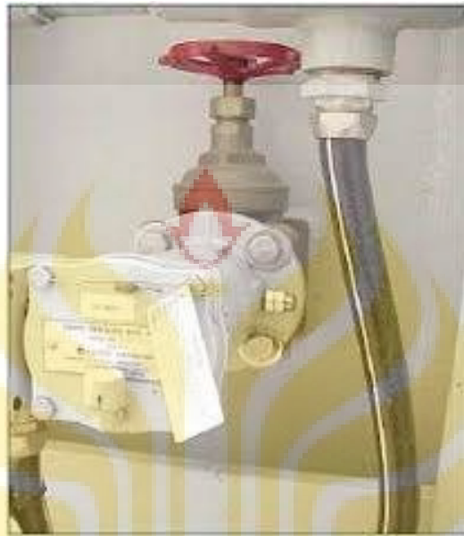
Gambar 11 Sudden Pressure Relay
