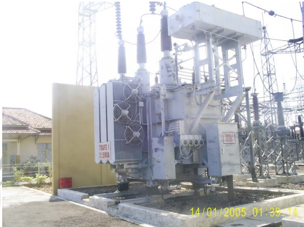
Gambar 3. Peralatan Arestor GI Sronдол 150 KV
