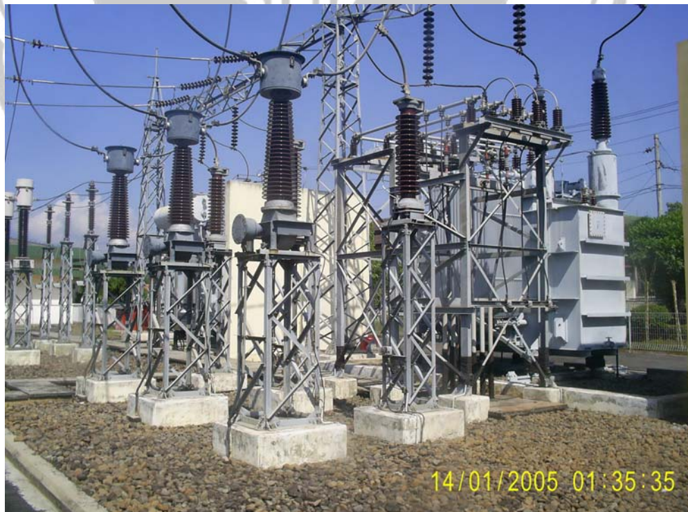
Gambar 3. Peralatan Arestor GI Sronдол 150 KV
