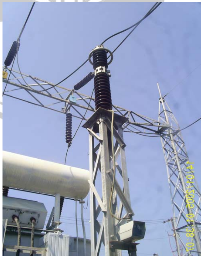
Gambar 5. Arester tipe X AR 170 A 1 / 162 GI Sronдол 150 KV
