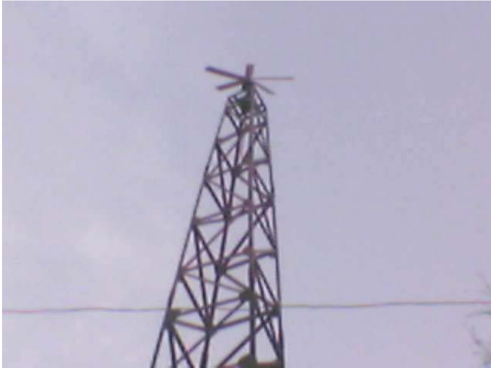
Gambar 15. Sesudah alternator dipasang
